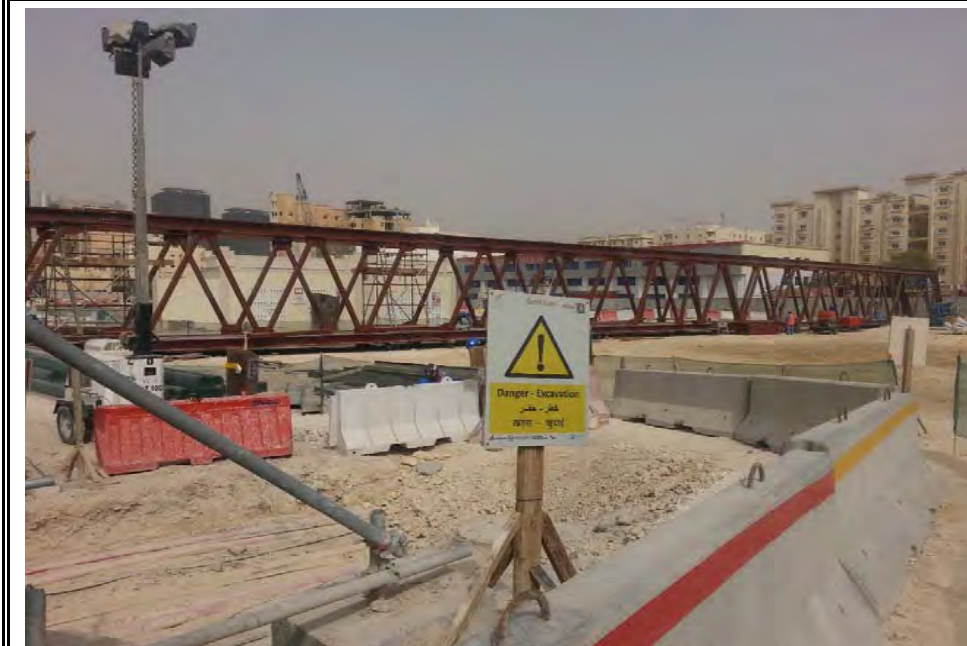
70M STEEL BRIDGE IN GOLD LINE METRO PROJECT
