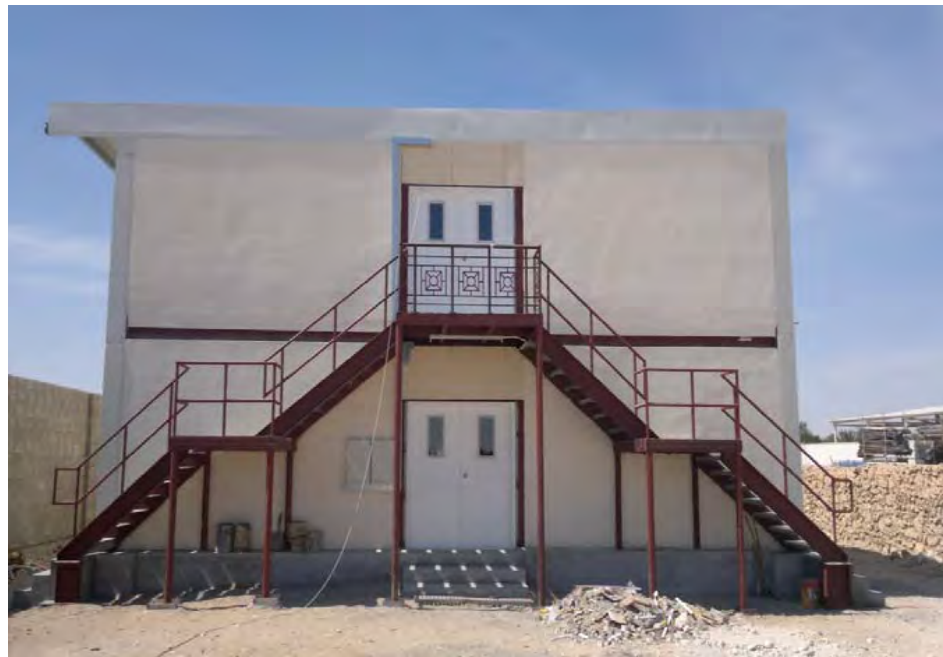
CHURCH COMMUNITY CENTER, DECORATIVE HANDRAIL
